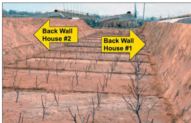
Fig. 7. Foreground view of solar lean-to greenhouse with sunken floor before superstructure and side-walls established. Typical, established, simple, south-facing, solar lean-to greenhouses in the background in Changli, Hebei province, P.R. China in April, 2010. (Photo by D.R. Layne).
