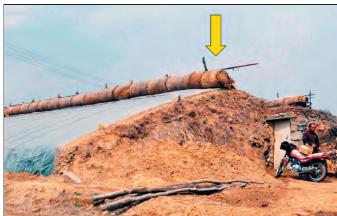
Fig. 8. Typical, simple, south-facing, solar lean-to greenhouse with sunken floor growing white-fleshed peaches in Dalian, Liaoning province, P.R. China in April 2010. Side and back walls are made of earth. Crop advancement is 30-90 days using this system. Note non-transparent insulation blanket (straw mat; see arrow) rolled up at top of house. (Photo by D.R. Layne).
